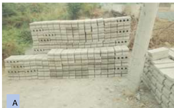
Figure 2.6 (A, B & C) Hand-made bricks /Sun-dried bricks (Byone-brick) are used as construction of buildings.
